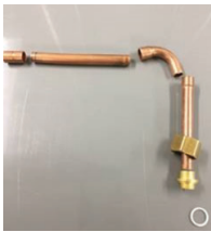
Fig. 16 — Braze Street Elbow
